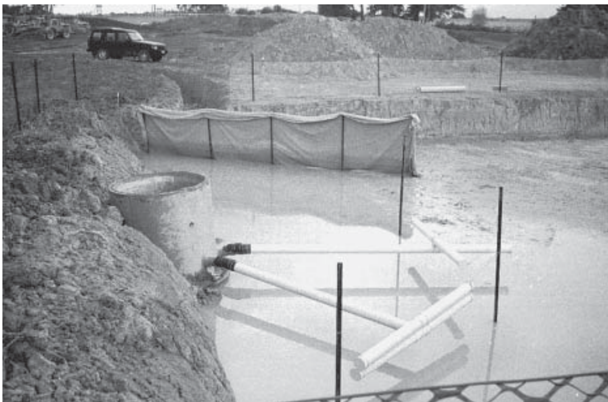
Plate 2.1.2 Sediment Retention Pond Showing Baffle to Lengthen Flowpath and Create Correct Length:Width Ratio
