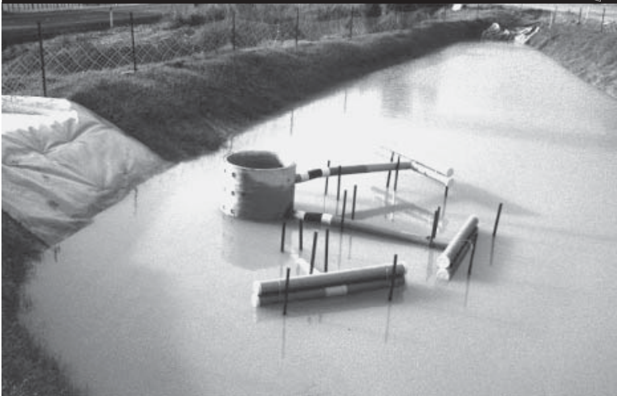
Plate 2.1.1 Sediment Retention Pond Showing Decant Systems
